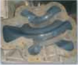
Casing after repair.
